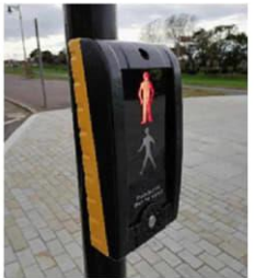
Typical Example of a pedestrian signal push button
